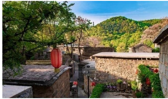
Fig. 2. Xiuwu County Xicun Township after renovation
